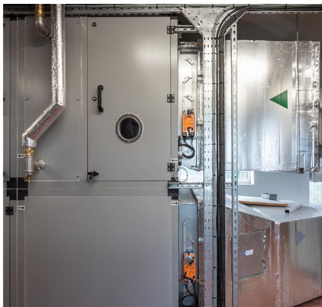
Across all cleanroom-classified areas of the new Chemotherapy Aseptic Suite and CT/ATMP Aseptic Facilities, the environment will have a strict tolerance of the temperature control as well as upper humidity limits being maintained for occupancy comfort. The Grade C areas are maintained at  $19^{\circ}\text{C} \pm 2^{\circ}\text{C}$  whilst the Grade D rooms are maintained at  $19.5^{\circ}\text{C} \pm 1.5^{\circ}\text{C}$ , both areas are controlled with an upper limit of 55% relative humidity.
